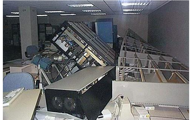
Abb. 2.21.2 > Umgekippte Computerracks
