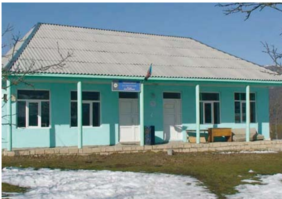
Primary school in Sis, Azerbaijan, after renovation in May 2009
