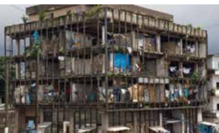
Abandoned office building in Monrovia, housing urban internally displaced persons
